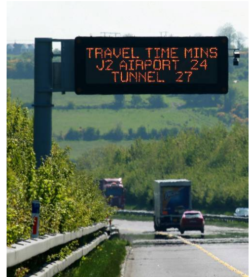
Figure 3.3: Typical LED VMS (Continuous Matrix)
